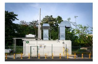
This site in Anasco, Puerto Rico is utilizing a 2G system with the generating capacity of 240 kW electrical and 367 kW thermal. This unit is generating both the heat and power for a local resort using propane as the source of fuel. It is fully containerized with Island Mode for resiliency and continuous operation during blackouts or natural disasters (hurricane) The system is rated to withstand tropical winds and seismic activity.
