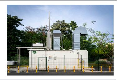
This beach resort in Añasco, Puerto Rico, uses a 2G patruus 400 with a generating capacity of 240 kW electrical and 367 kW thermal. This unit generates heat and power for the resort, using propane as the fuel source. This unit is fully containerized with Island Mode for built-in resiliency and continuity during a blackout or natural disaster (hurricane), and rated to withstand tropical winds and seismic activity.
