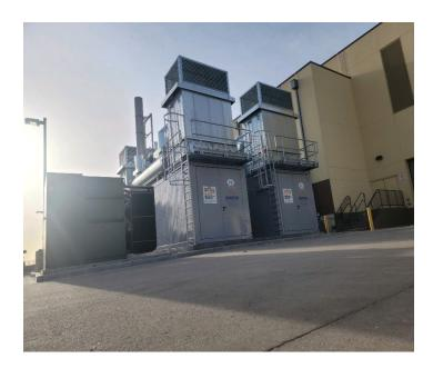
4.0 MW of installed electric capacity, with two 2.0 MW generators operating at 73.2% efficiency
